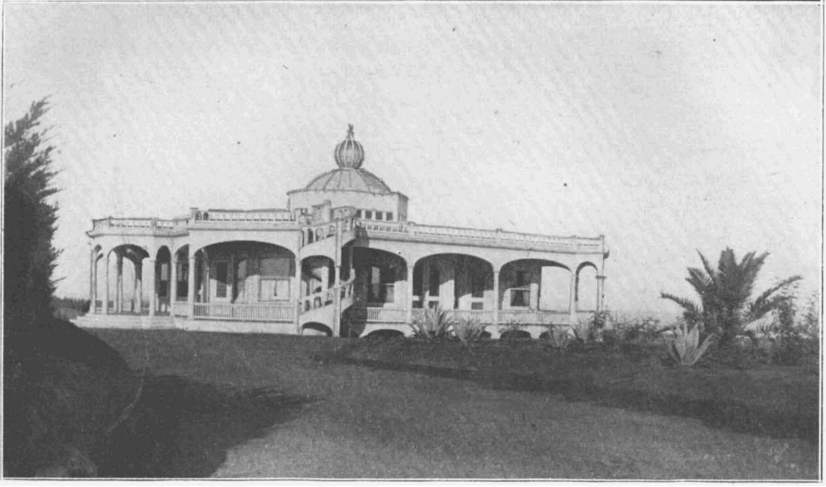
YERBA SANTA CLIFFS, STUDENTS' GROUP HOUSE NO. 1, POINT LOMA
